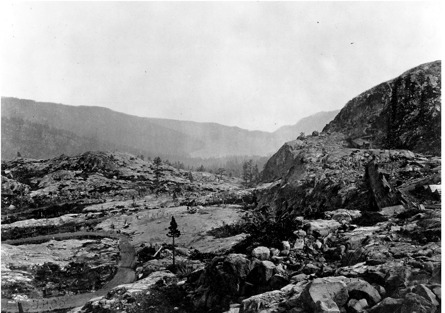
Donner Pass in the late 1860s. Note Central Pacific Railroad construction tents on far right of photo and the Chinese walls prior to back filling. The Dutch Flat Road is on the left. Donner Lake is barely visible in the center background.
