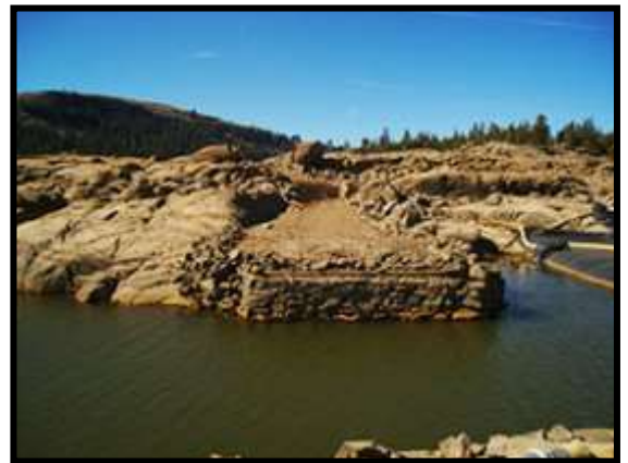
Alpine Highway Bridge Abutment
